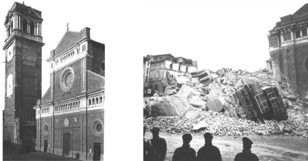
Fig. 7 The collapse of the historical civic tower of Pavia in 1989 (Binda, 2008)
