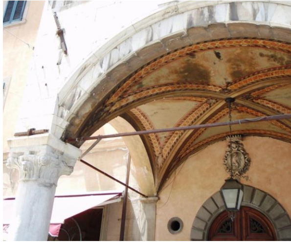
Fig. 14 Presence of horizontal prestressing steel bars in masonry vaulted structures
