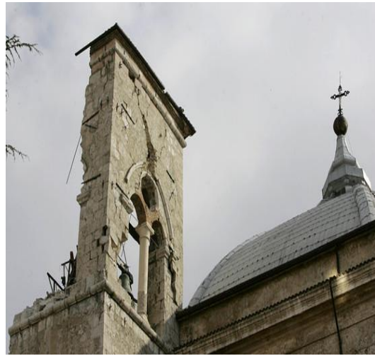
Fig. 3 San Bernardino church in original conditions and observed damage after the 6.3 magnitude earthquake of L'Aquila, Italy on April 6 th 2009
