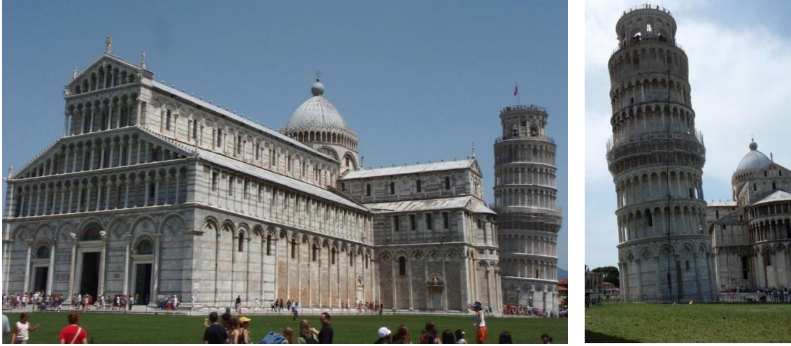
Fig. 8 General view of the leaning tower of Pisa, Italy
